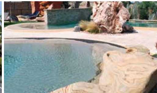
PISCINE SWIMMING POOLS
